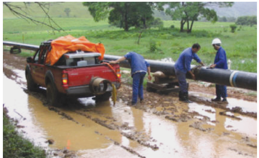
Figure 7. Inspections were carried out in difficult terrain and under arduous conditions
